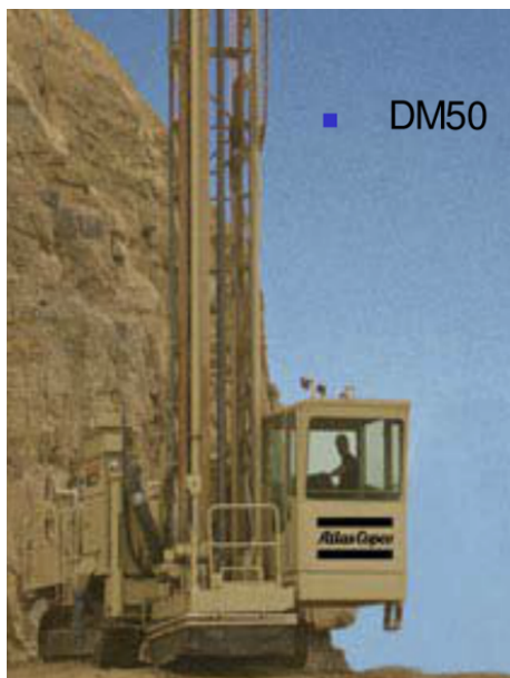
(a) Rotary drilling rig
